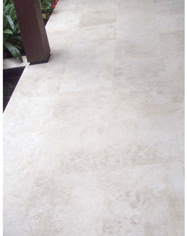
Limestone after cleaning with Skavenja™
